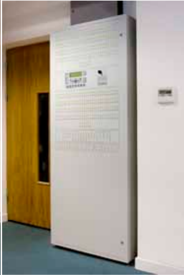
◀ Bespoke Fire Alarm Control Panel housed in a special compact enclosure to suit customers building layout.
